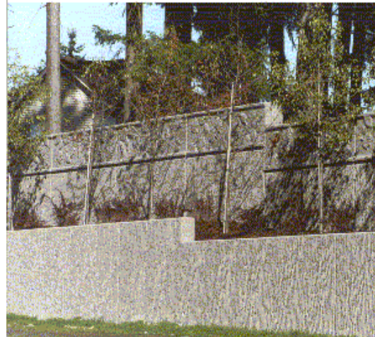
Exhibit 4 – Top of Noise Wall Steps Mirrored with Retaining Wall
