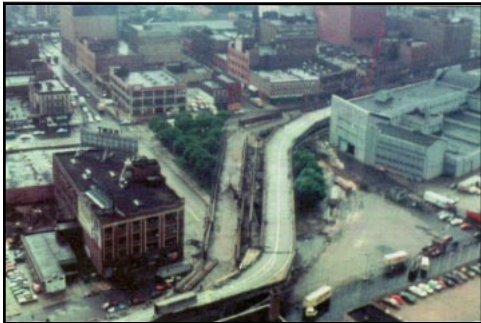
Section of collapsed West Side Highway in 1972.
