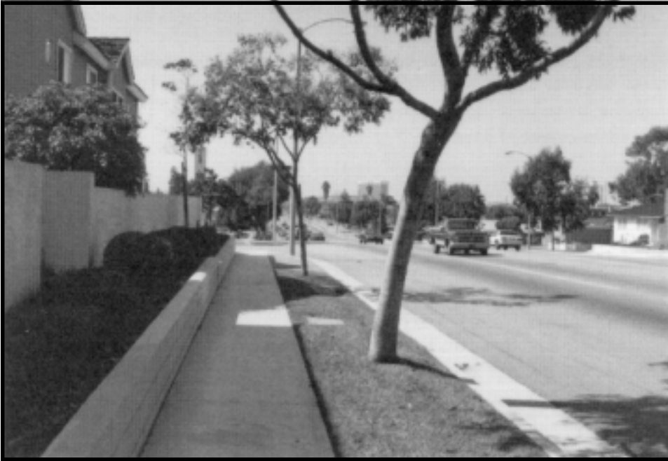
Plant materials and retaining wall.
