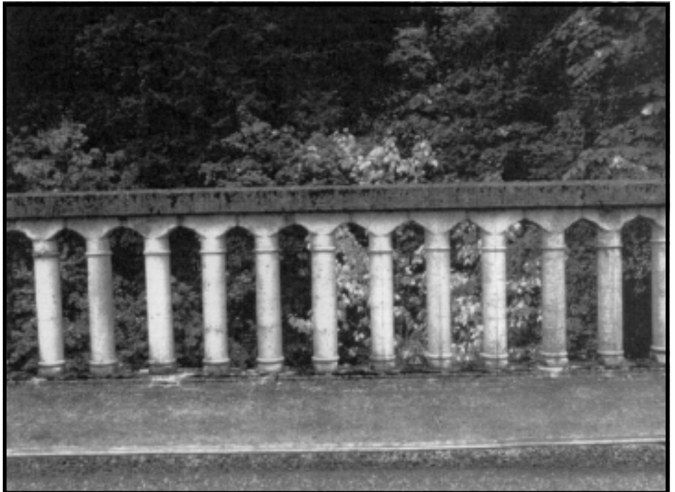
Spindle railing after restoration on the Young's Creek Bridge.
