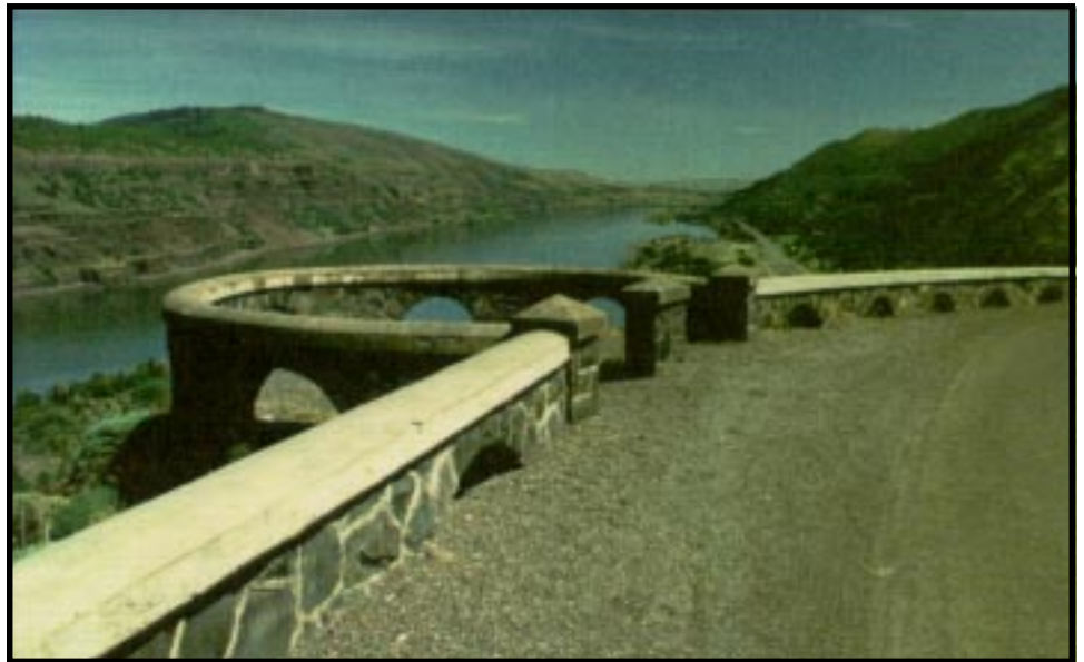
Typical overlook area along the highway.
