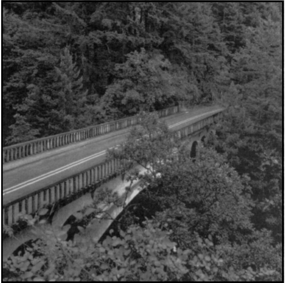
Young's Creek (Shepards Dell) Bridge after restoration.
