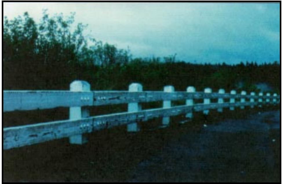
Newly installed steel-backed wooden guardrail.
