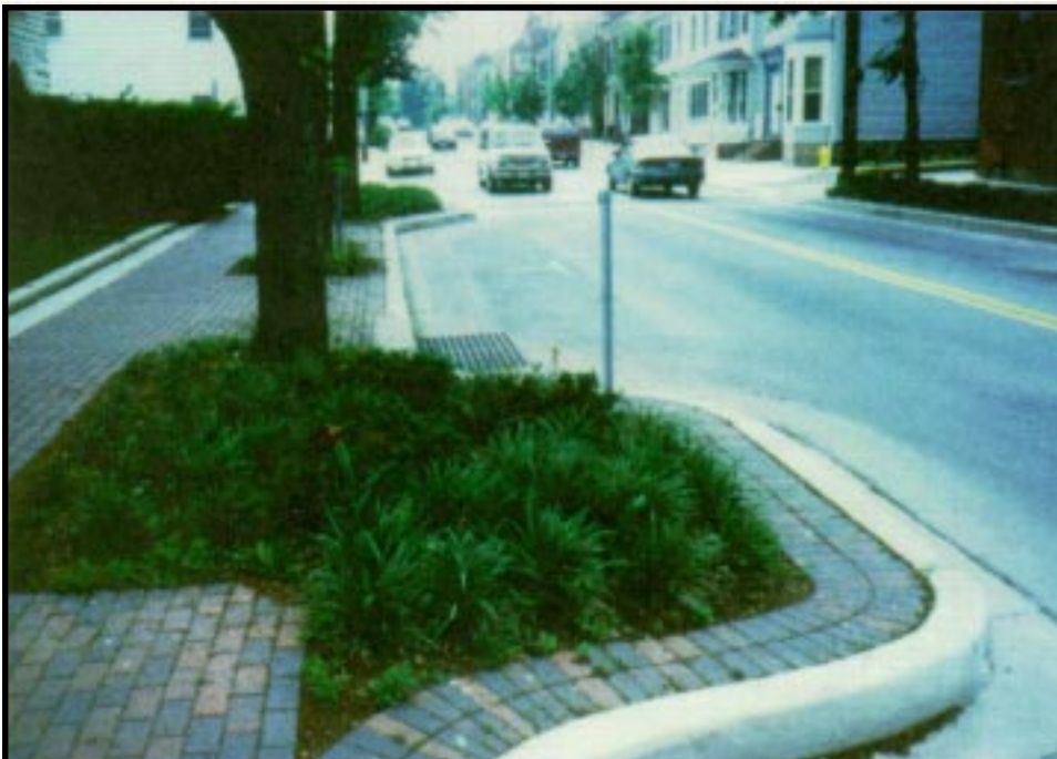
An area of extended curbing interlocks-an extensive area of low plantings with concrete pavers shaped like brick
