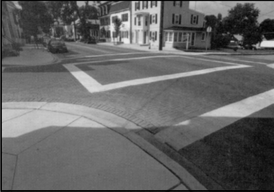
A crosswalk's well-defined rectangle contrasts with circular pavement-level corners. At left, the sidewalk has been widened to meet the outer pedestrian walkway border.
