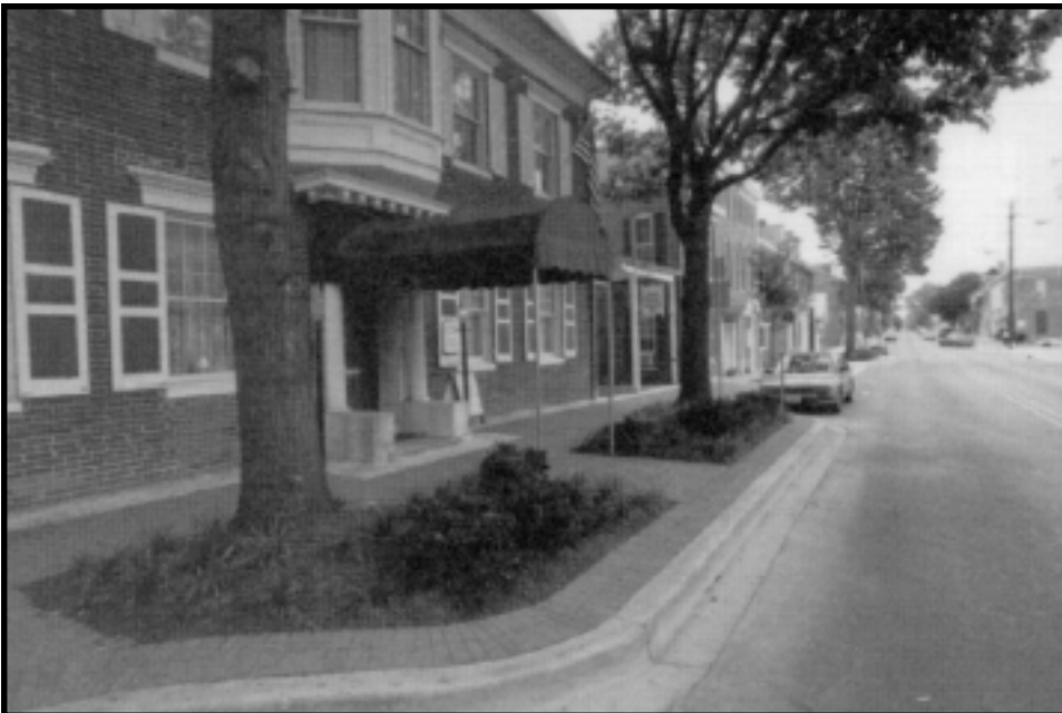
Extended curbings take on a variety of patterns, here highlighting a projecting entrance bay and awning. Note how the concrete curbing and building border form continuous lines into the distance.
