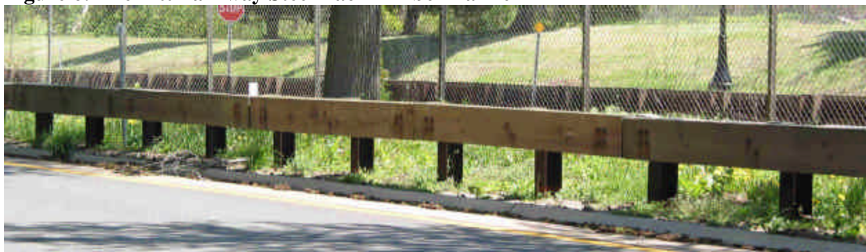
Figure 6: Merritt Parkway Steel Back Timber Barrier
