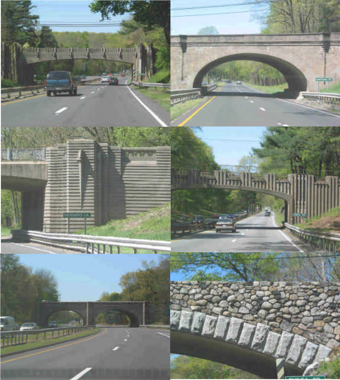
Figure 2: A Selection of Bridges on the Merritt Parkway
