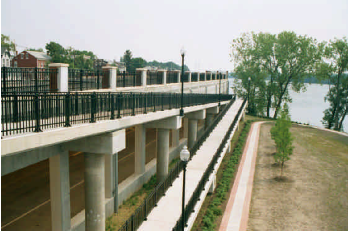
E.9 North end of tunnel.
