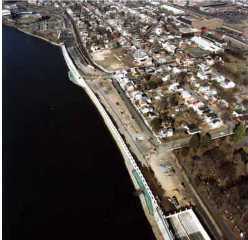
E.7 Completed tunnel project. Park on deck has not been constructed.
