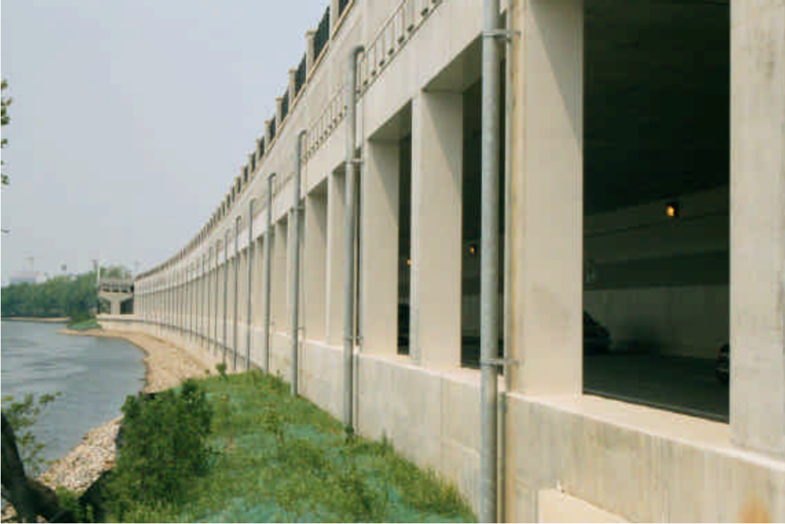
E.13 View of Route 29 tunnel from shoreline.
