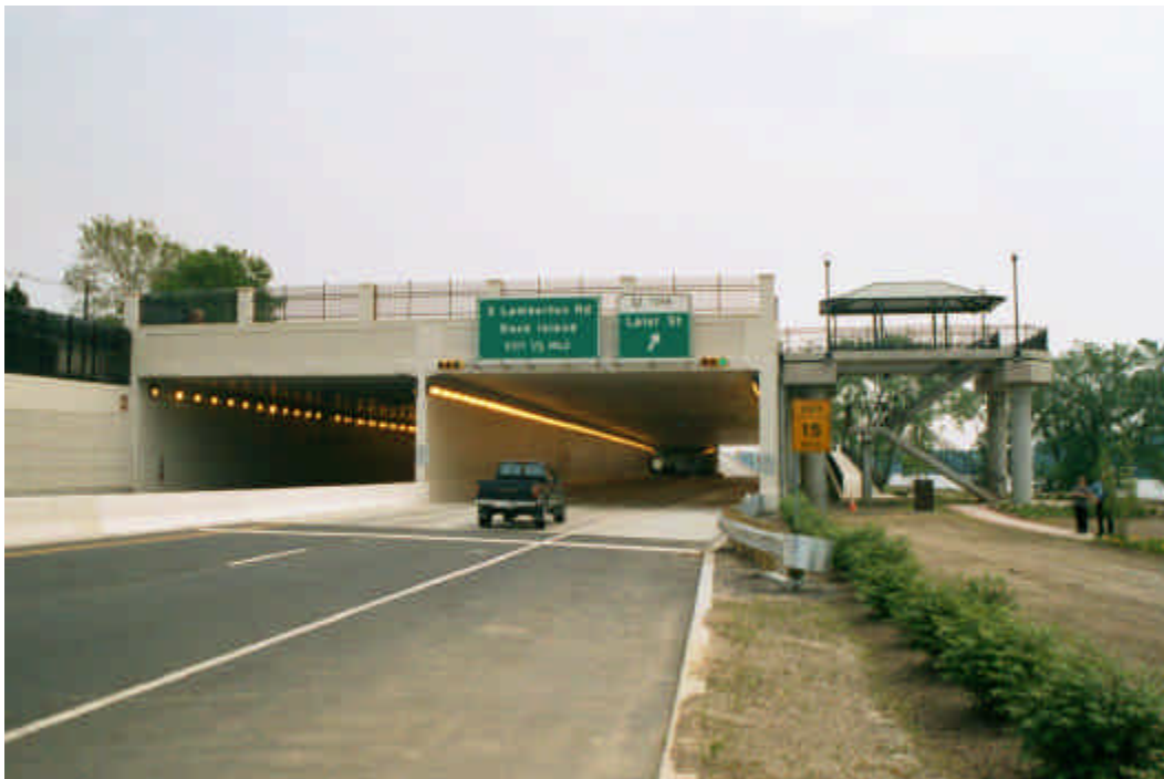
E.8 Tunnel entrance from north.
