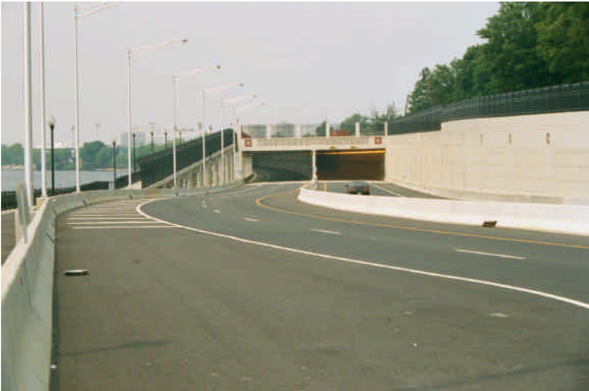
E.14 Entrance to tunnel from south.
