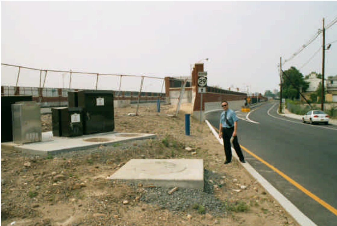
E.12 Entrance to tunnel at mid-section. Note utility boxes that will need to be moved or hidden.
