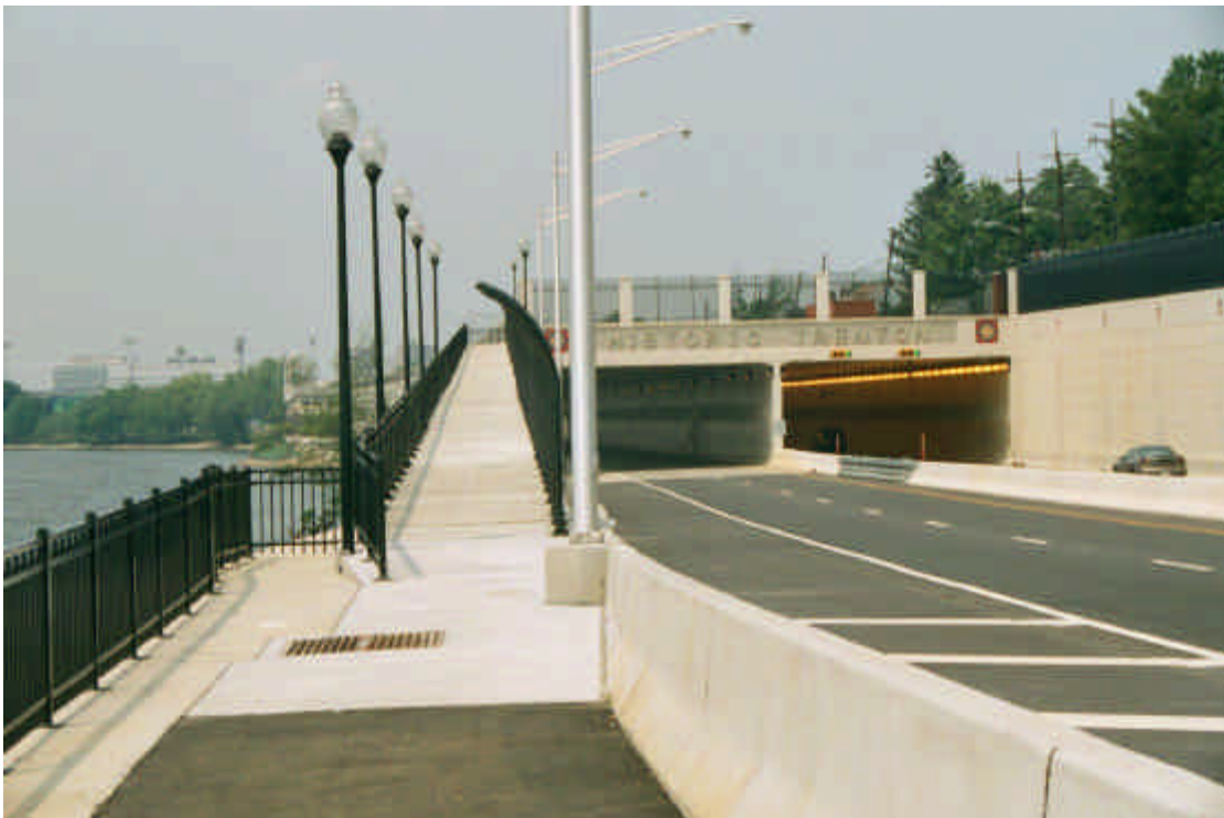
E.16 View of walkway next to south tunnel entrance. Safety fencing at right of walkway was to match that on other side of road but contractor did not put in footings adequate to support the fencing that was specified.
