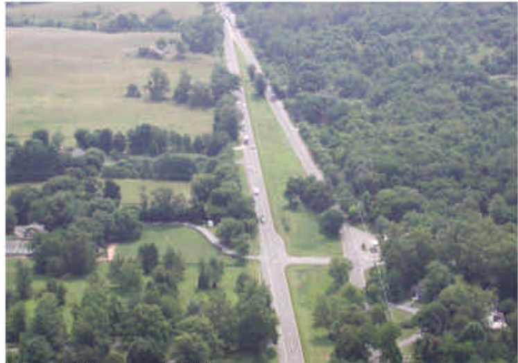
4 lane section, looking east towards Middleburg.
