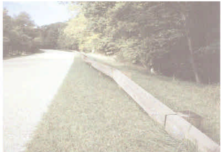
Example of steel-backed timber guardrails
