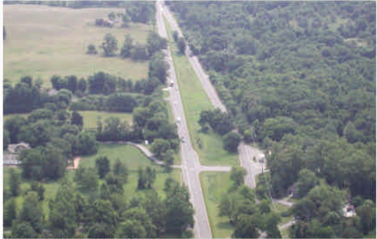
4-lane section of Route 50 west of Middleburg
