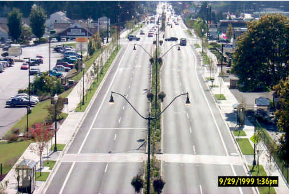
Figure 4. Bridgeport Way after, south view
