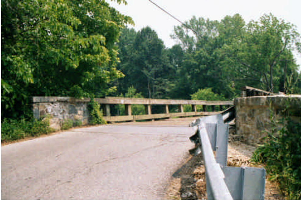
B.7 Smiths Bridge from West approach.
