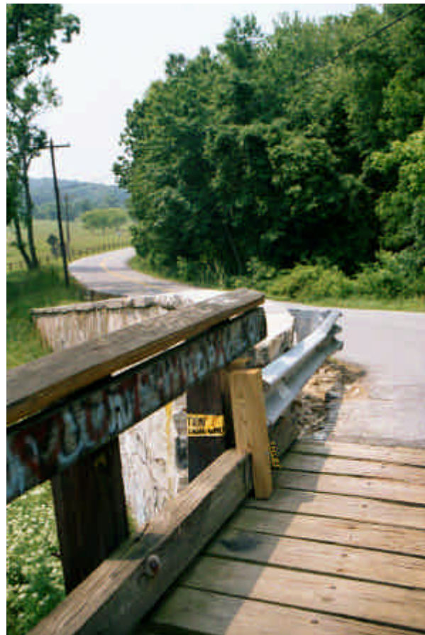
B.8 Close up of Smiths Bridge at west approach.
