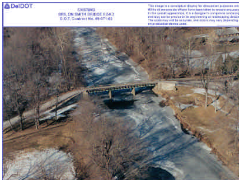
B.2 Aerial view of existing Smiths Bridge.
