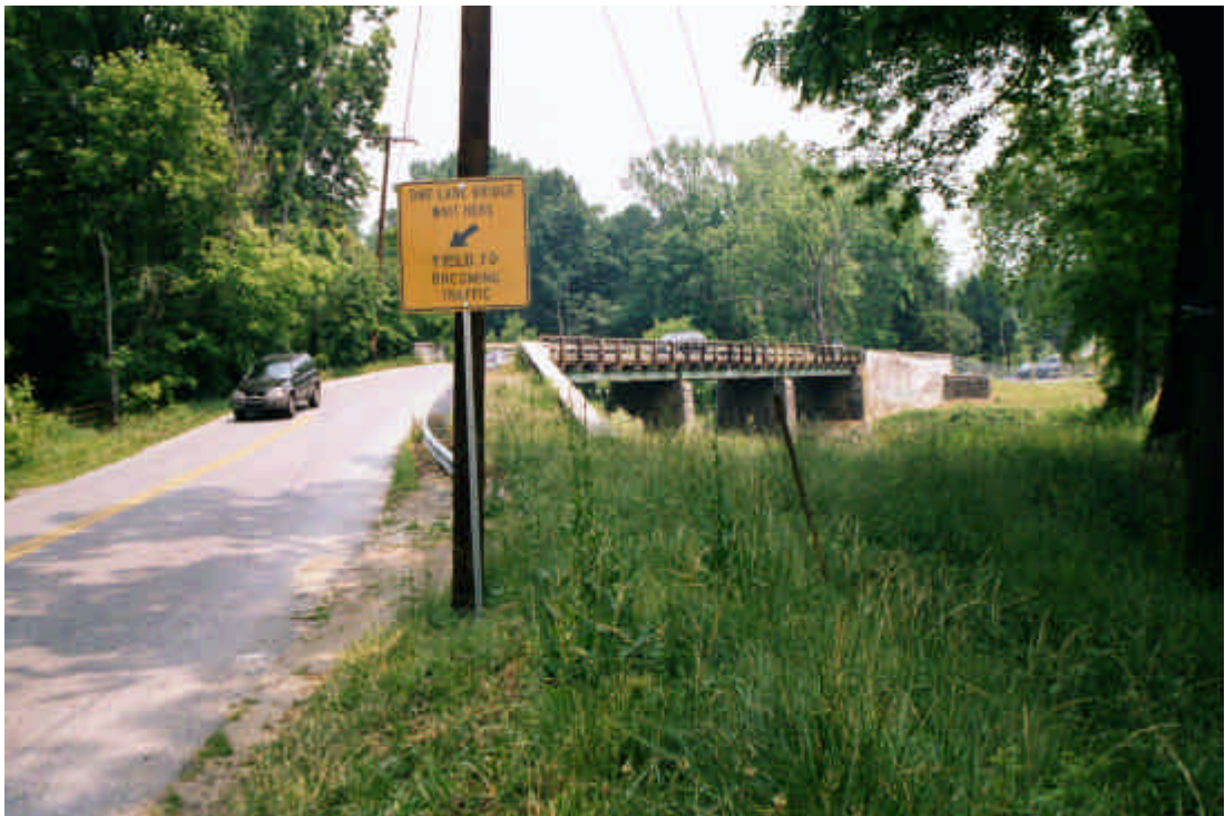
B.6 Smiths Bridge from west approach.
