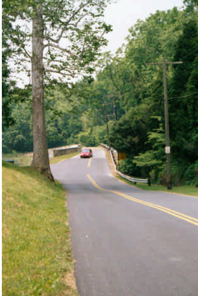
B.1 Smiths Bridge from the east approach.
