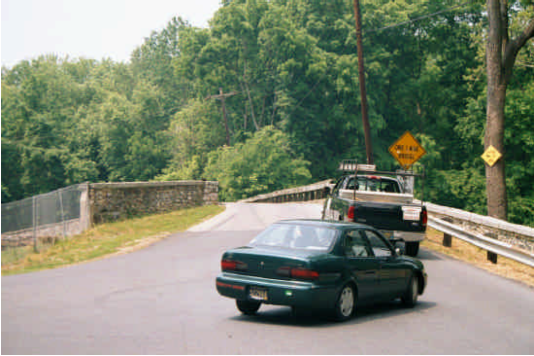
B.5 Smiths Bridge from east approach.
