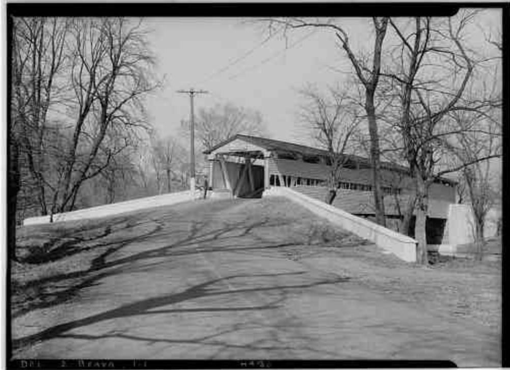
B.9 HABS Photo of Smiths Bridge constructed in 1839. Photo was taken from east approach in 1939.
