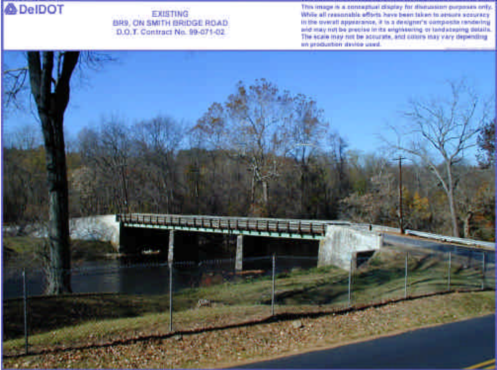
B.3 Side view of existing Smiths Bridge
