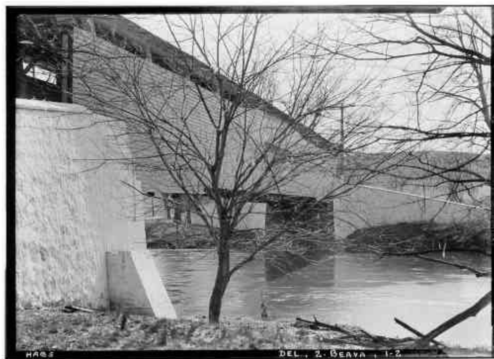
B.10 HABS photo of Smiths Bridge with side view taken in 1939.
