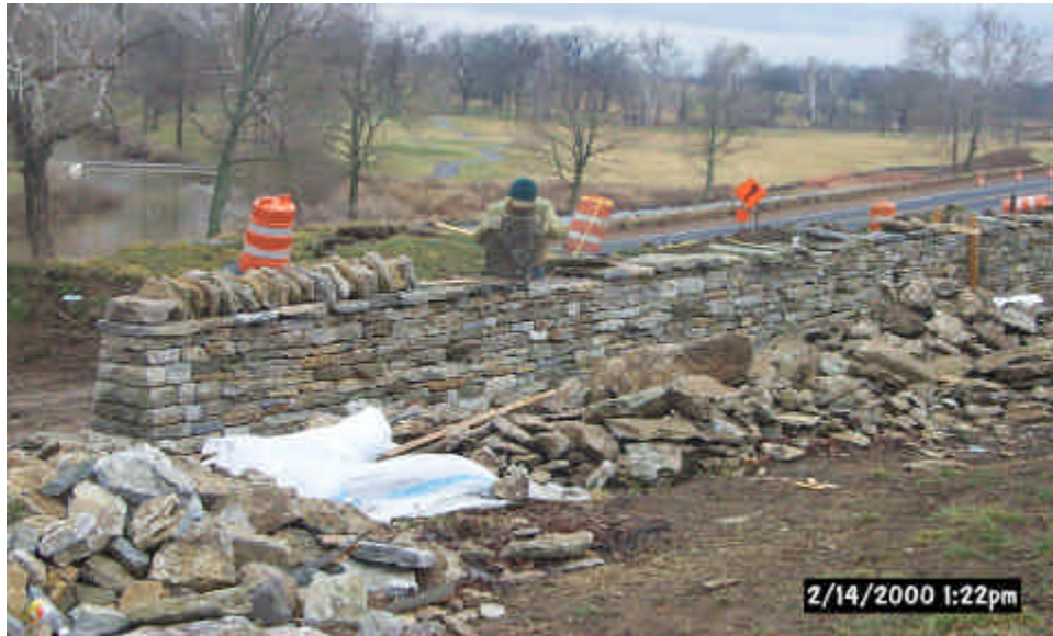
If not, stonewalls were dismantled and rebuilt
