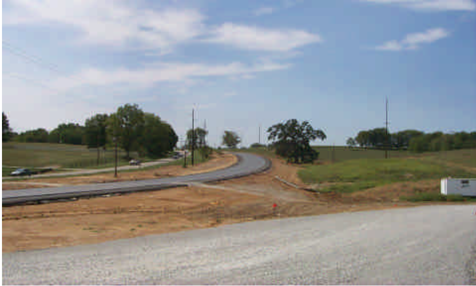
The roadway alignment was adjusted to selectively keep, or replace, specific tree species
