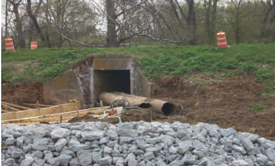
A water channel change combining multiple water channels performed to allow for a single culvert installation to minimize and control erosion
