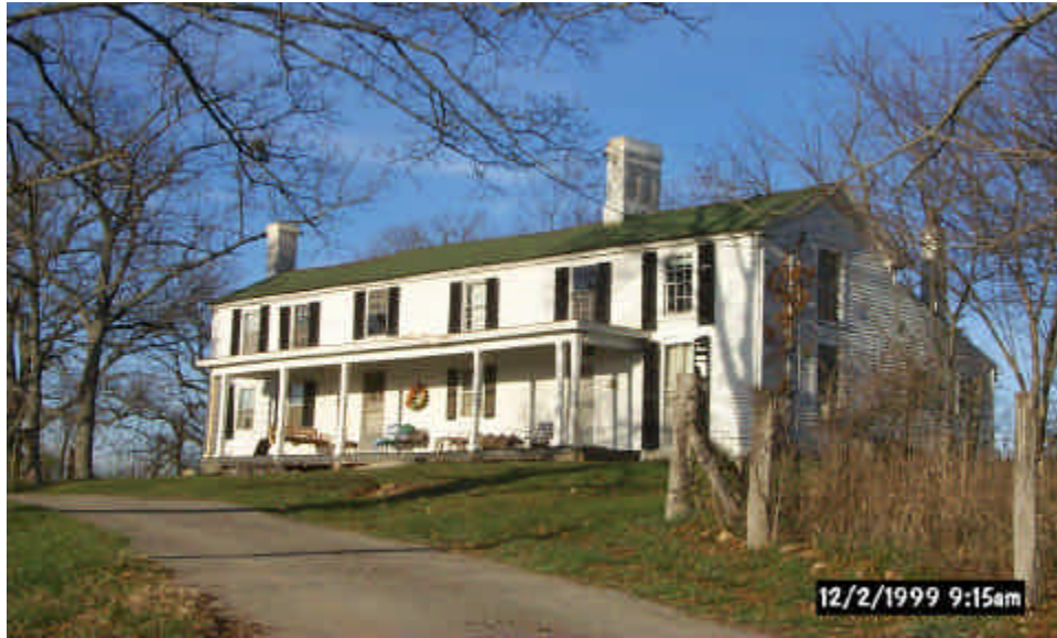
A house on the Historic Registry was refurbished as an interpretive center
