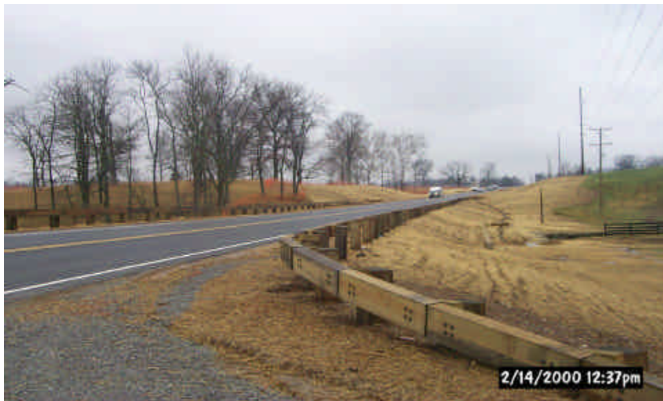
Steel-backed timber guardrail was used to provide driver safety while giving strong consideration to aesthetics
