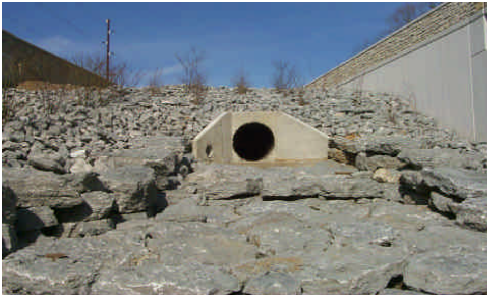
Scupper slab erosion control technique was used at the Paris bridge
