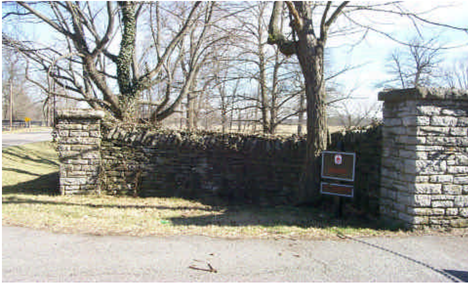
Historic signature entrances to the horse farms were avoided by roadway alignment or rebuilt to original form
