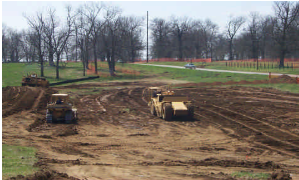
The original topsoil, Marnie silt loam, was stripped, stockpiled and returned to the original 1 to 1½ foot thickness
