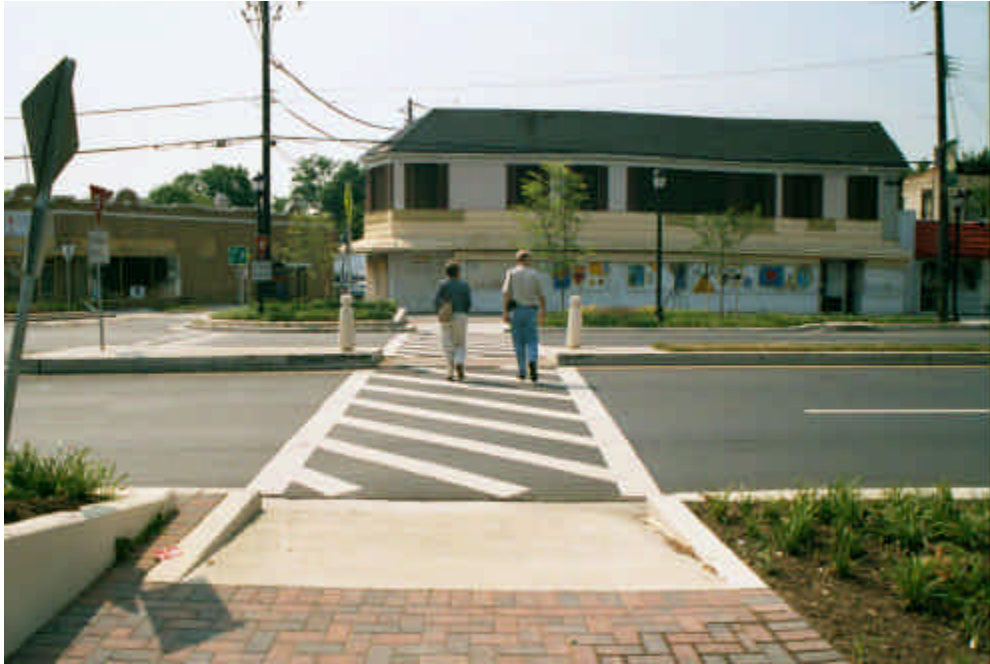
C.11 Non-signalized crosswalk at south side of roundabout allows for easier and safer crossing than previously.
