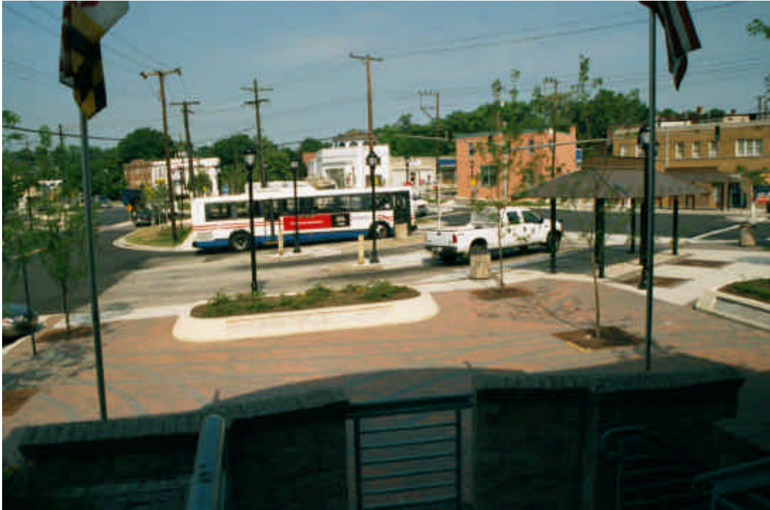
C.7 Mount Rainier roundabout after photo taken from steps of City Hall showing bus holding lanes, bus shelters, and paving patterns to reflect historic trolley lines.
