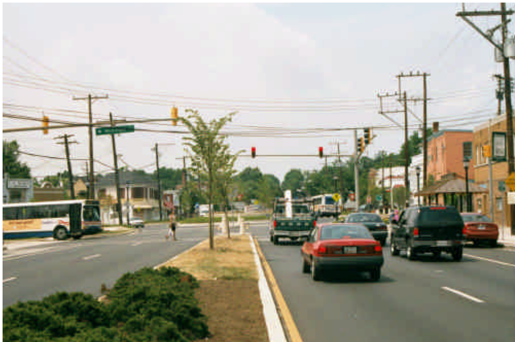
C.10 Signalized crosswalk at north side of roundabout allows buses to reenter traffic and pedestrians to cross street.
