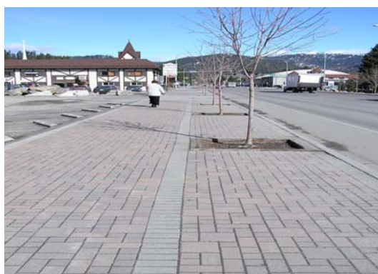
Exhibit 3 – Finished Patterned Sidewalk
