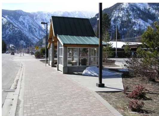
Exhibit 2 – Finished Sidewalk and Bus Shelter
