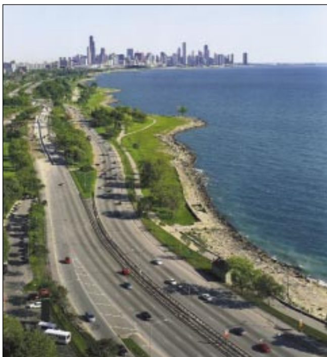
South Lake Shore Drive is one of Chicago's primary commuter routes, carrying more than 100,000 vehicles a day. It is also a popular scenic drive alongside Lake Michigan. State and local transportation agencies balanced these demands by using a context-sensitive reconstruction plan that not only improved the roadway but enhanced the neighborhood.
