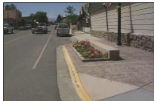
Improved parking along the main street was one of the many benefits citizens gained from the project. (All photos courtesy of Montana DOT.)
