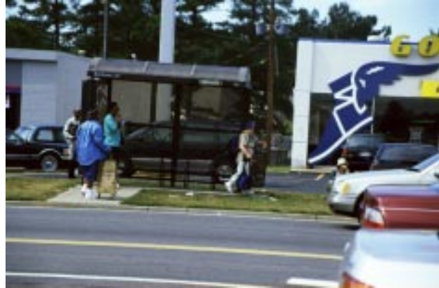
Undesirable bus stop placement.
